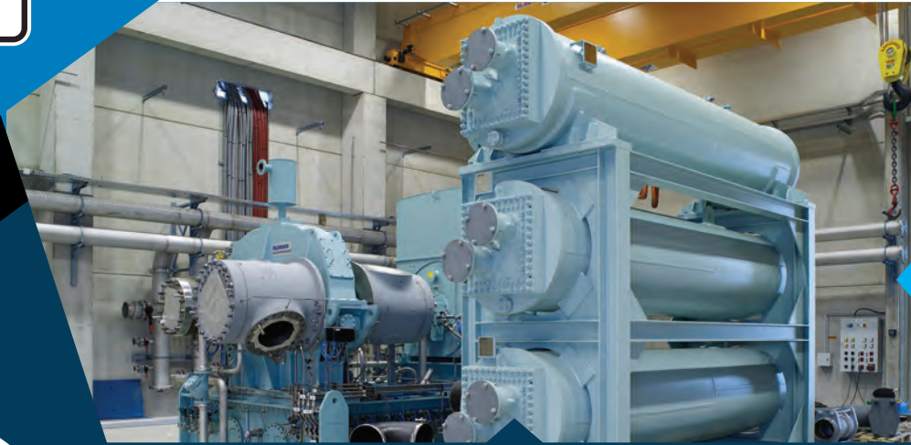
Compander with water cooling system for marine applications
